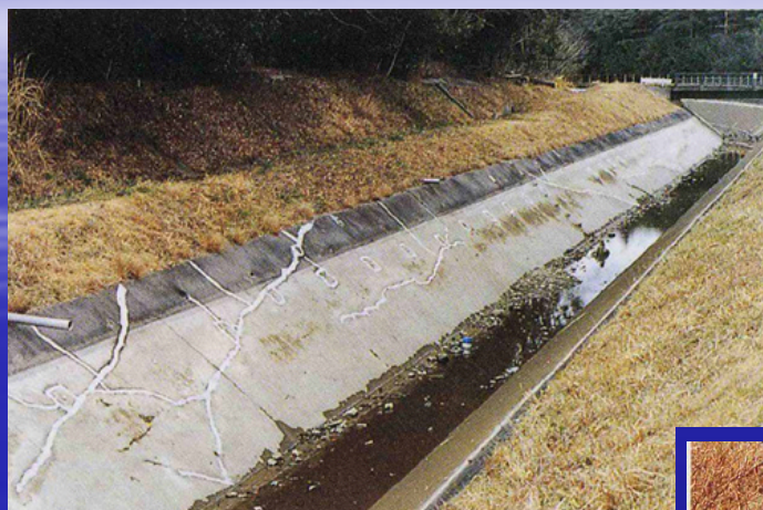
Cracked Lining
